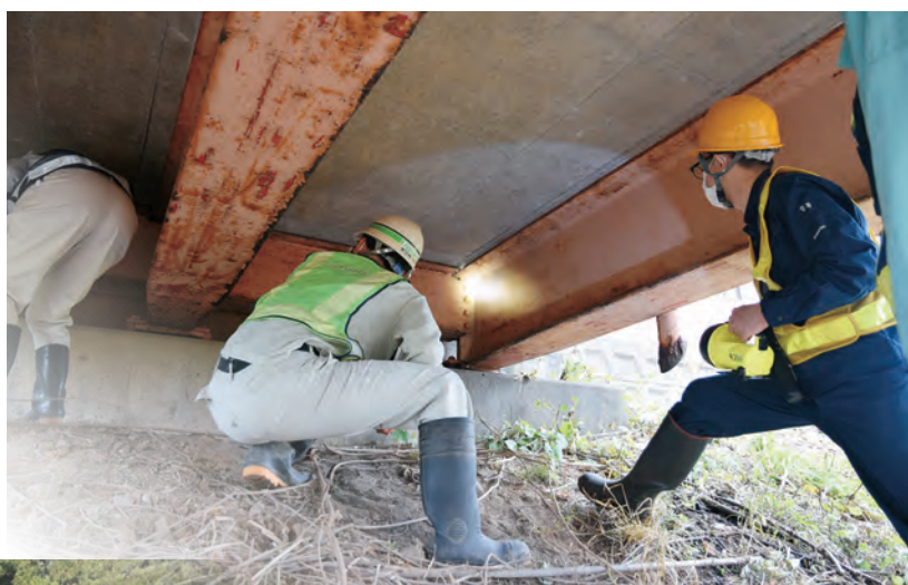
実構造物での実習 Practical training with actual structures
